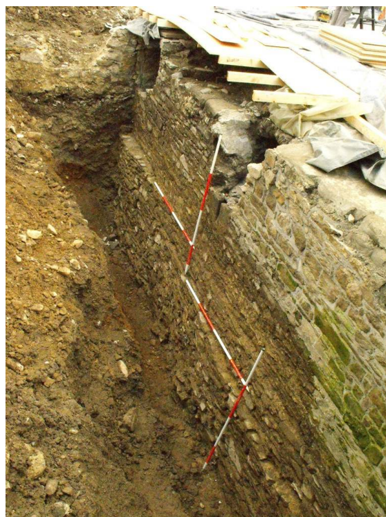
Exterior footing at west wall during excavation, 2011
