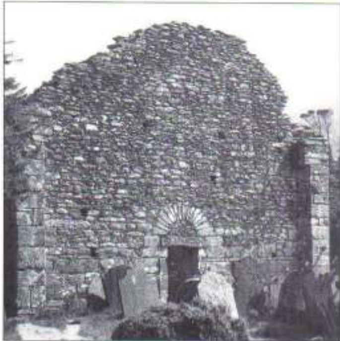
Pl. 1. The west end of the cathedral at Glendalough. Note the antae with a wide section at the top and the large stones in the lower course of the wall. (Photo O.P.W.)
